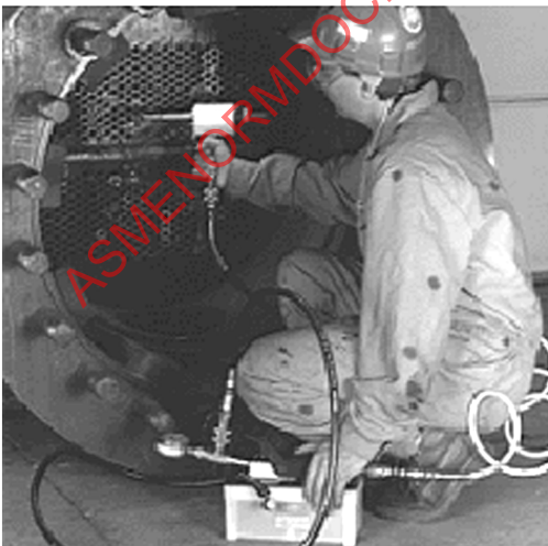
Figure 312-4.2-3 Typical Installation of Mechanical Fit Tube Plugs
