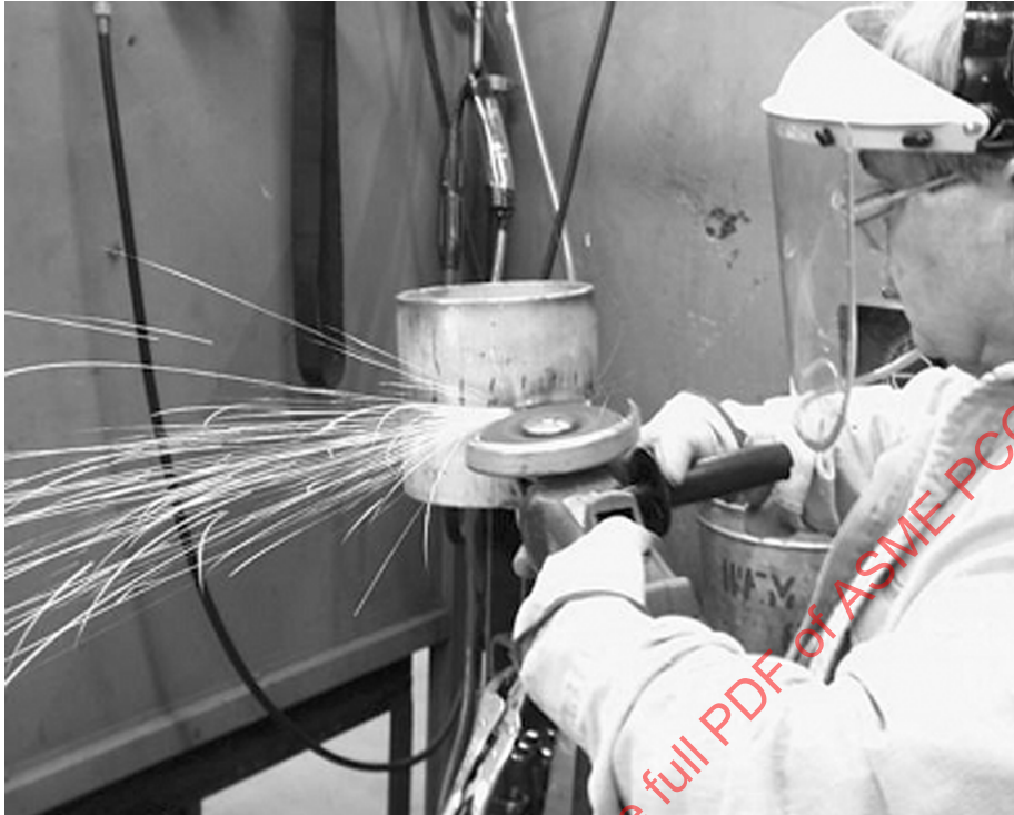
Figure 304-3.1-3 Grinding of Weld Flaw
