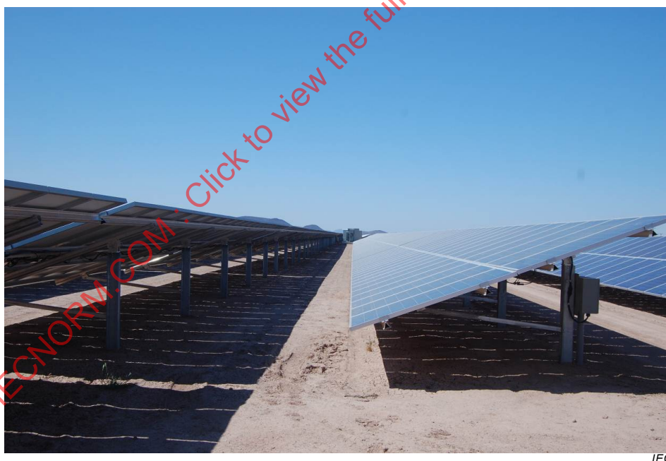
Figure 5 – Example power plant with fixed tilt array
