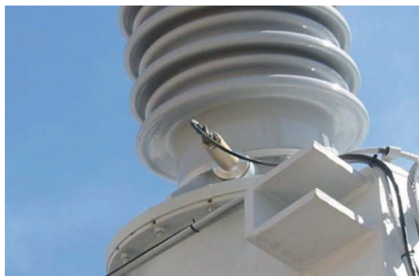
Figure 6 — Capacitive sensor mounted in bushing tap
