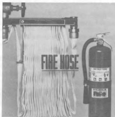
Figure 3-1(d) Semi-automatic hose rack assembly.
