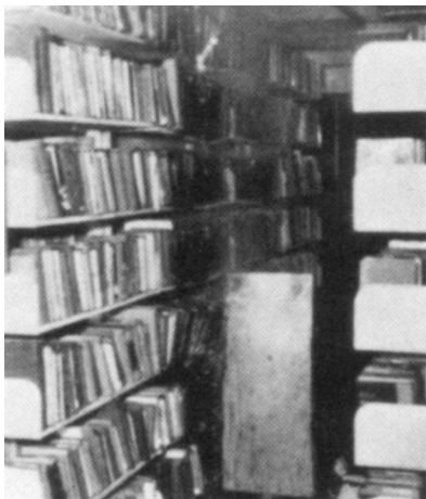
Figure J-2(e) After fire extinguishment by sprinklers; fire damage to books in only 10 percent of space.
