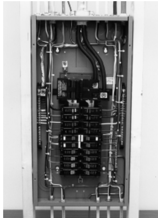
FIGURE 6.6(d) Circuit-breaker panel.
