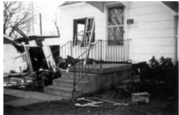
FIGURE 18.3.1 Low-order damage in a dwelling.
