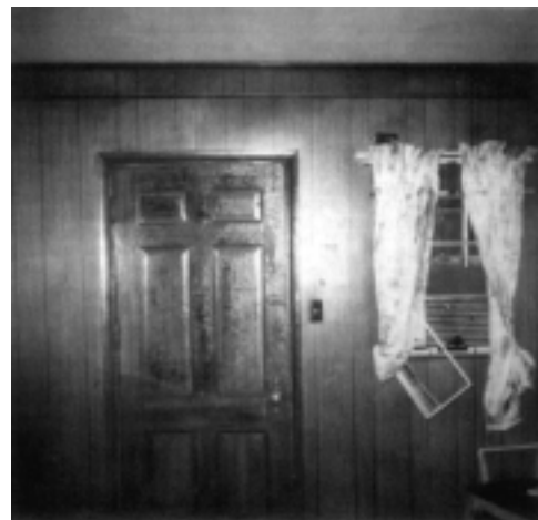
FIGURE 4.19.2 Blistering of varnish on door and slight scorching of draperies, the only indications of the natural gas flash fire.
