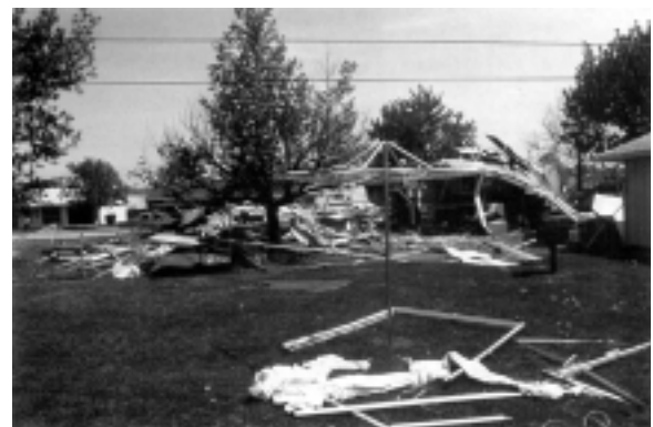
FIGURE 18.3.2 High-order damage shown by shattered and splintered remains of a four-bedroom house.
