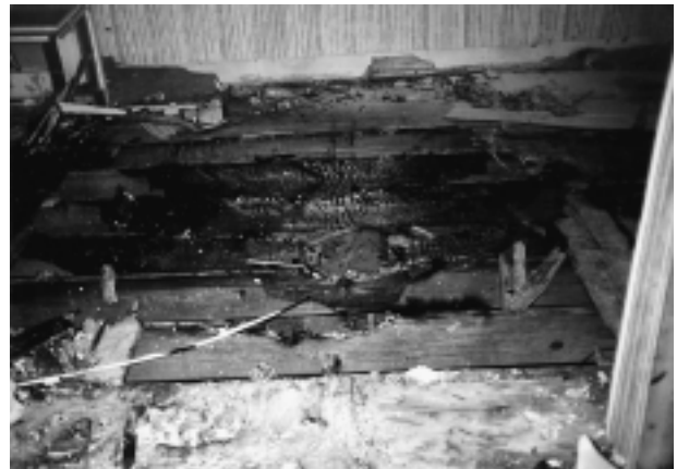
FIGURE 4.17.10 Saddle burn in a floor joist.
